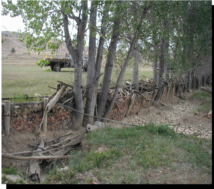
Flood Irrigation uses spreader dikes to capture CBM water and irrigate crops by spreading the runoff.
